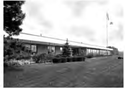
USA – Danaher Controls Gurnee, Illinois
